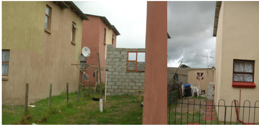
Figure 8 : Sakhasonke. Extension to building
