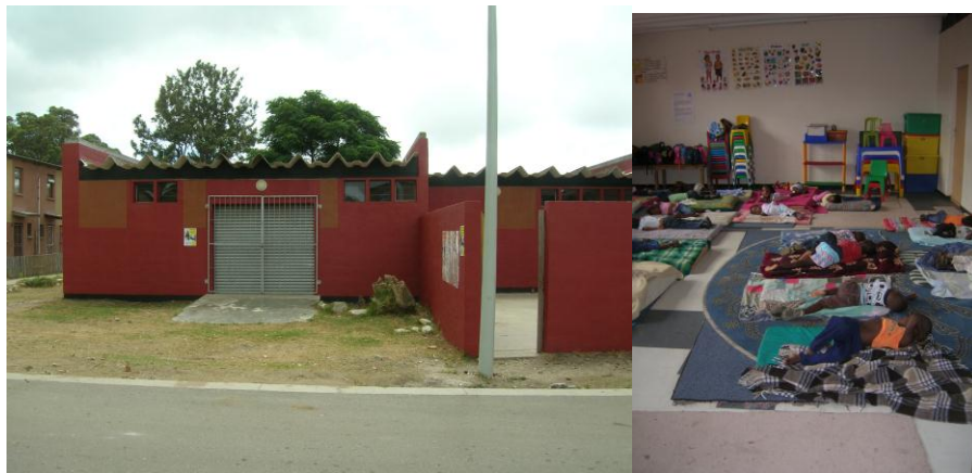
Figure 9 : Sakhasonke. Extension to building
